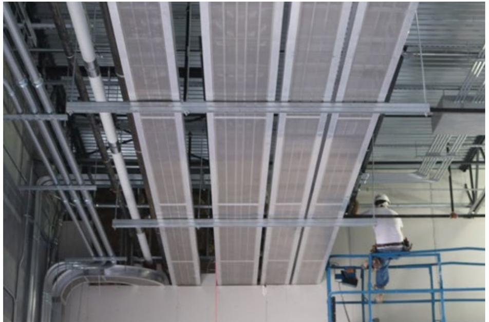
Worker pulling the cables of one system out of five running in the same facility to different laboratories.
