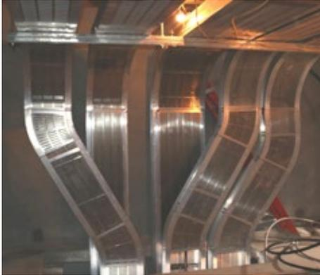
Transition from horizontal to vertical in a small opening
